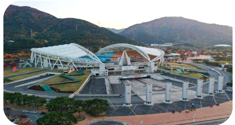
<Daegu Stadium - General View>
